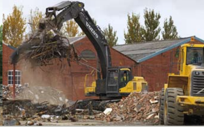
• Demolition excavators, wheel loaders — and more.
